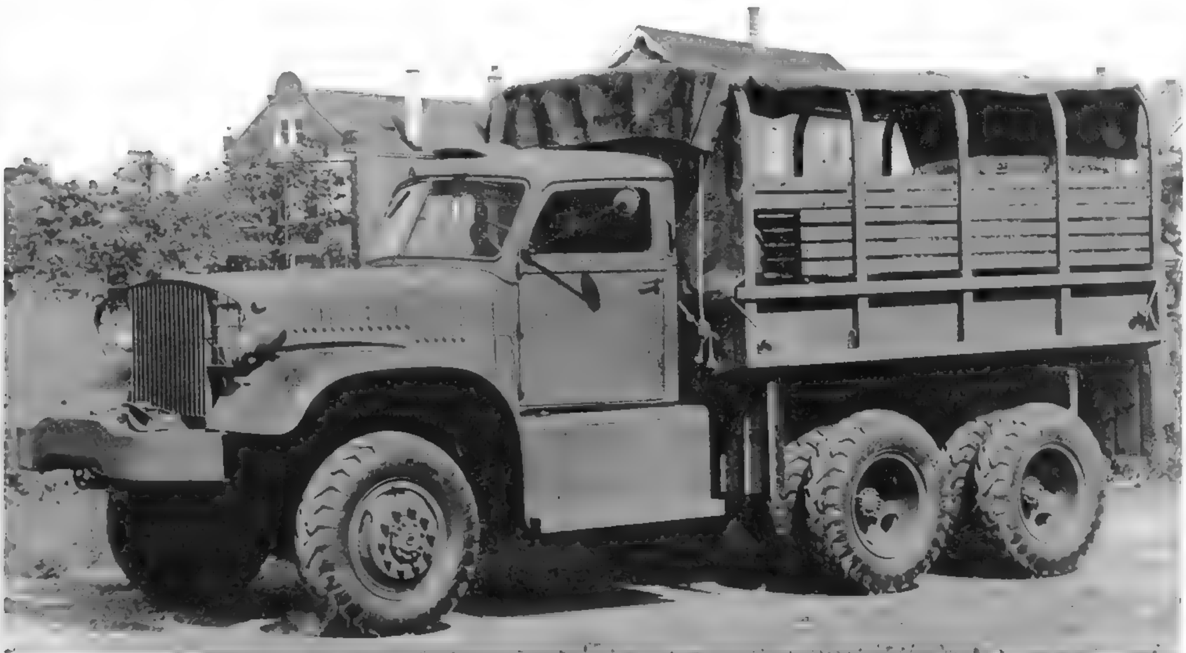
This photo shows the first truck in this series, the 4-ton 6x6 Diamond T Model 967. The identifying feature of this series is the brush guard that protects the radiator and headlights (Photo courtesy of the Patton Museum)
